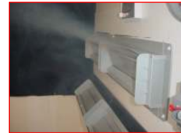
COLD SPOT NEAR LEAKING FAN SHUTTER
